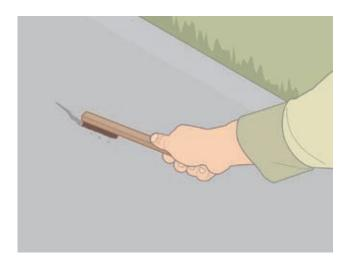
2. Clean out any dirt, organic matter, or concrete chips from the crack using a tool like a masonry brush, heavy paintbrush, or shop vacuum.
